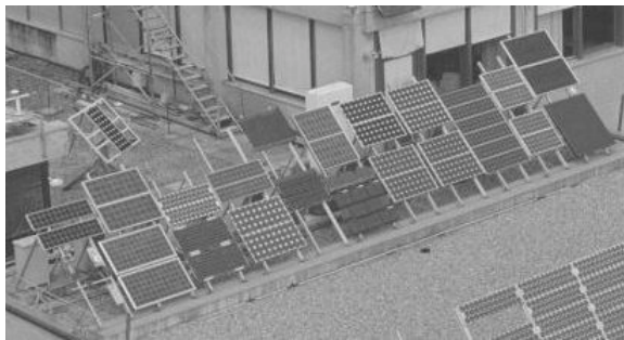
Figure 1: View of the LEEE-TISO test facility with the 17 modules under test.
